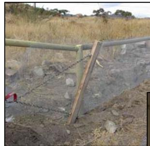
*A clamp for pulling the mesh and the lip at the base of the mesh to deter burrowing rodents.*
