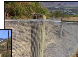
*The top edge of the mesh must be strengthened to prevent tearing.*
